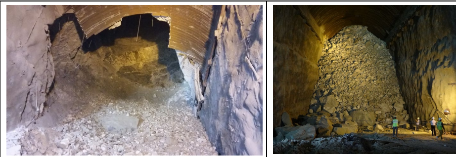
268 Fig. 26. There was an attempt to remove fallen rock (approx. 15,000 m 3 was 269 removed). Note the extra destruction of steel sets in the 'left' arch due to the 270 fault. A larger collapse subsequently occurred, shown on the right.
