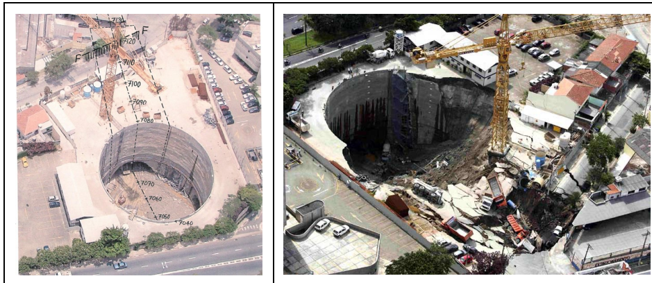
220 Fig. 18. The collapse of the Pinheiros Station cavern during construction. The 221 fatalities occurred along the small road (Rua Capri) seen on the right. 222
