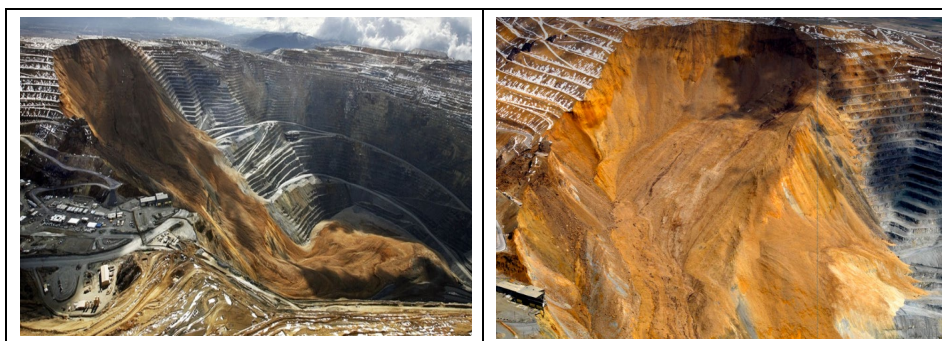
409 Fig. 40. A dramatic and record 70,000,000m 3 failure at Bingham Canyon 410 Mine in Utah. It measures 3km from crest to run-out toe. Some might assume 411 'circular' failure, but a 300-400m long fault plane was involved.
