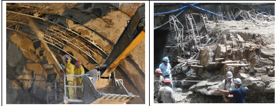
Fig. 21. Before and after. Lattice girders of 32mm x 25mm x 25mm capacity appear to have limited strength when confronted with a large concentrated vertical load. Designers are usually assuming a rare evenly distributed load.
